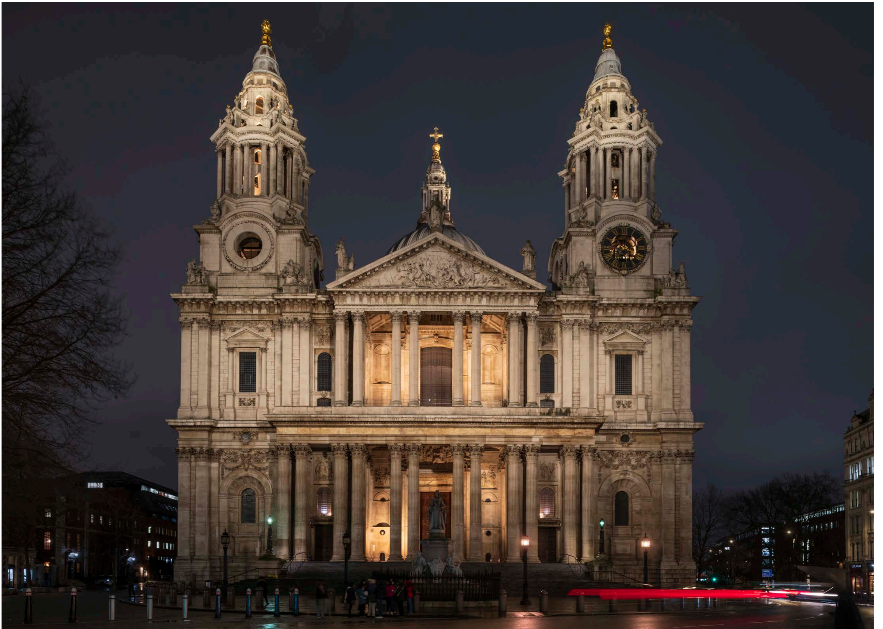
Lighting trial: West façade view from Ludgate Hill, early evening scene.
